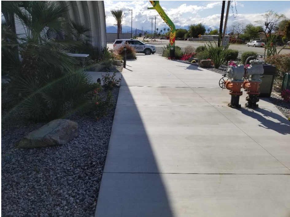
Front Entry is missing “Bicycle Racks”
