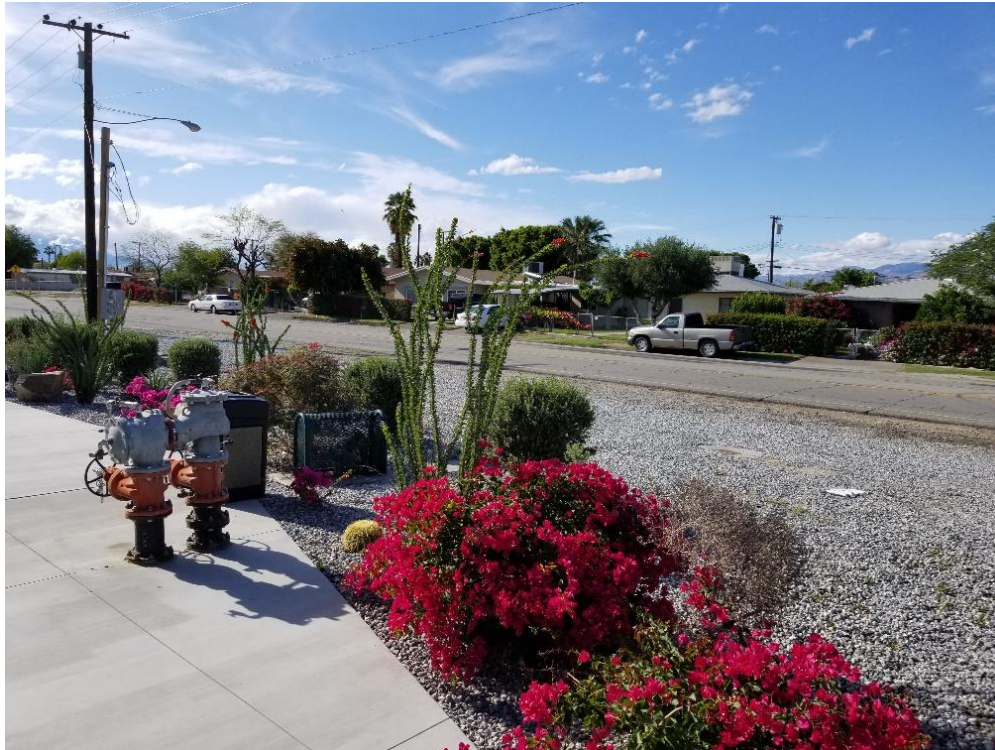
Landscaping along Avenue 48 is missing the required "Perimeter Fencing"
